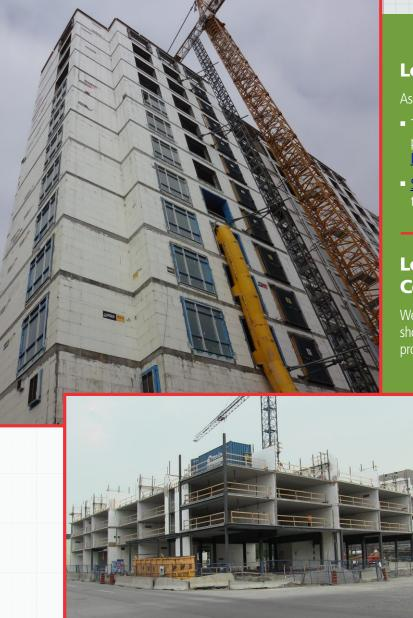
Logix ICF is easy to learn and is accessible to framers, masons and concrete contractors.
