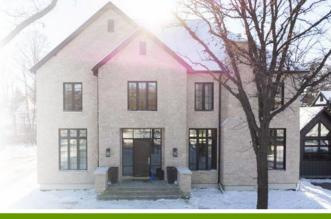
The design of this house matches the timeless and iconic design of stately surrounding manors. Built with 4" core Logix ICFs, this design features 26 corners and two levels of 11' walls over a full height 8" basement.
