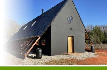
This design concepts has roots in the ancient Viking Longhouse and it creates an ideal space for passive cooling and heating techniques. This A-frame structure creates great thermal mass while the roof system, which overhangs each side by 9', provides lots of space for covered porches and greenhouses.
