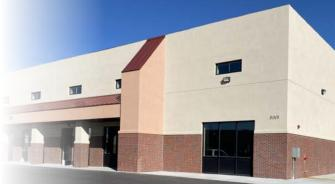
This commercial building design featured tall Logix ICF walls supporting a steel truss EPDM roof system.
