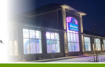
This is a fairly intricate structural design that was complicated by the number of massive windows, a lack of load-bearing interior walls and the tall 14' exterior walls. The design also featured arched openings and a stone veneer.
