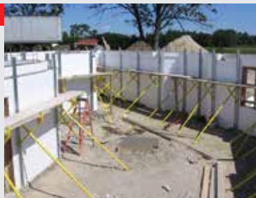
4 Brace the wall
