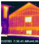
Thermal image of a conventionally built home
