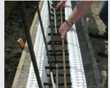
3 Place the rebar
