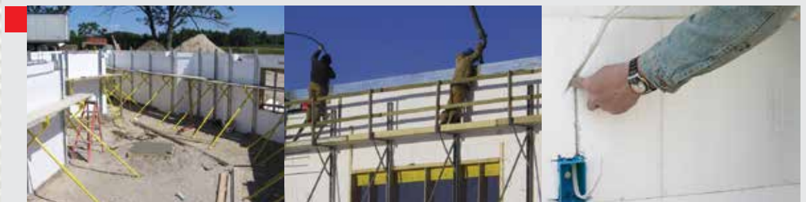
4 Brace the wall
