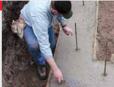
1 Prepare the job site
