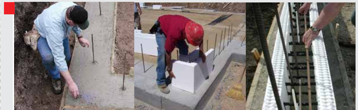
1 Prepare the job site
