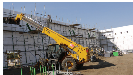
Logix High Performance Tall Walls (in progress)
