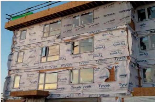
*Figure 2.5 Poor House Wrap Installation*
