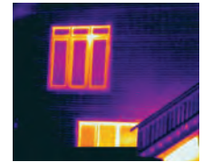
Thermal image of a Logix XtraComfort building
