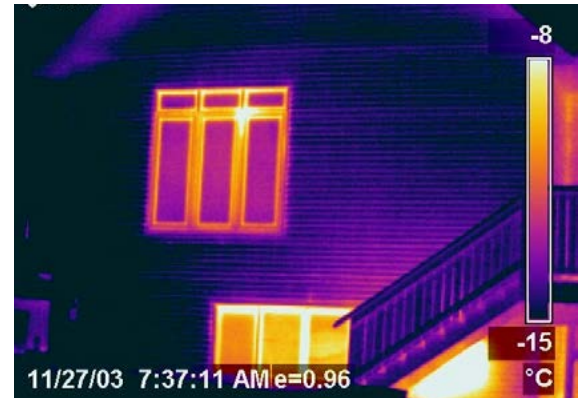
Logix ICF Thermal Image
