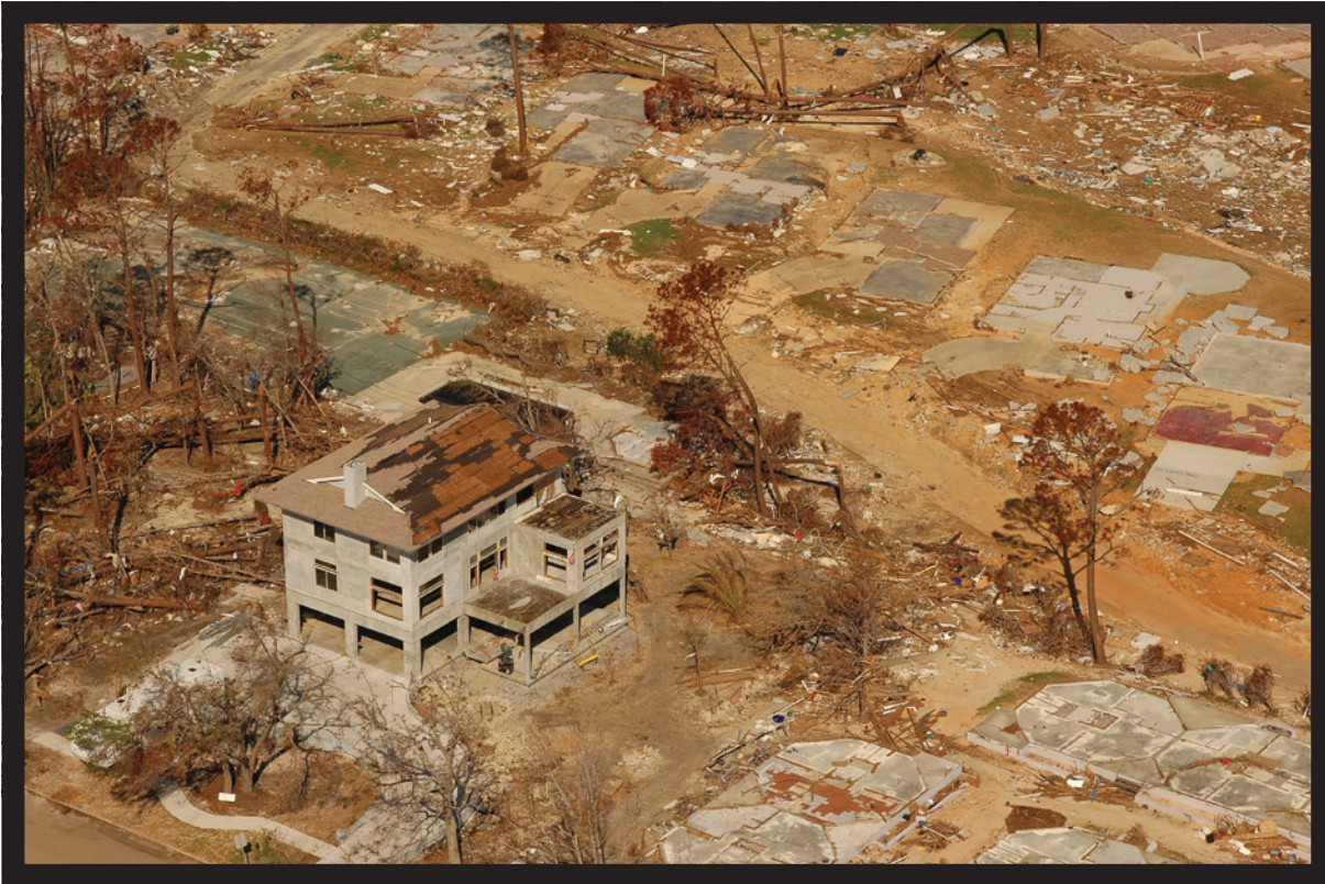
Actual ICF-Built Home That Survived Katrina
